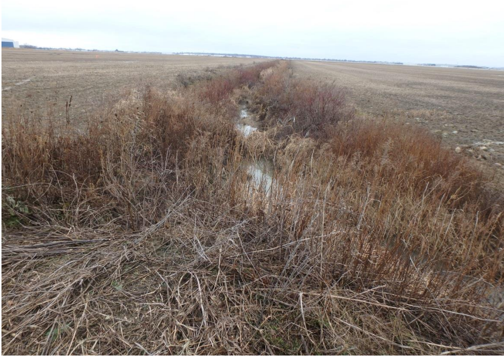
Photo 7 – Lappan Drain, Looking West
