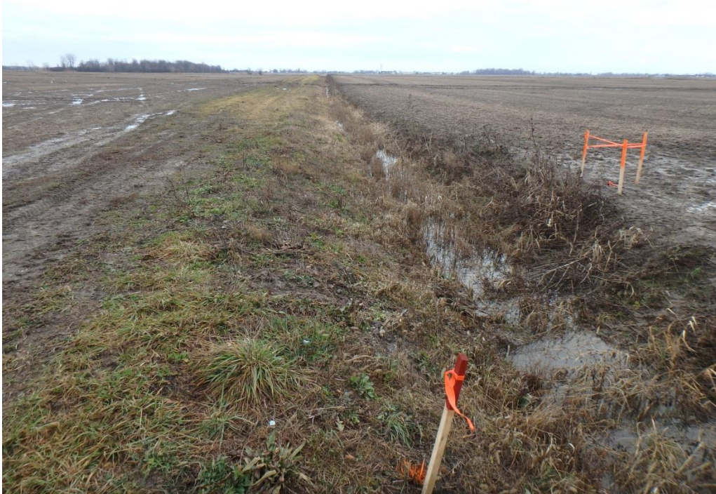
Photo 9 – Ditch South of Runway, Looking South
