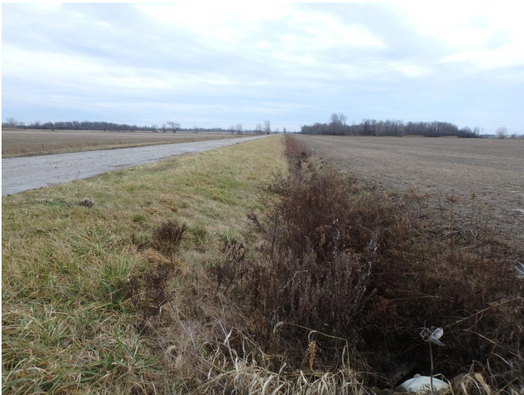
Photo 12 – Jefferson Boulevard Roadside Ditch, Looking South
