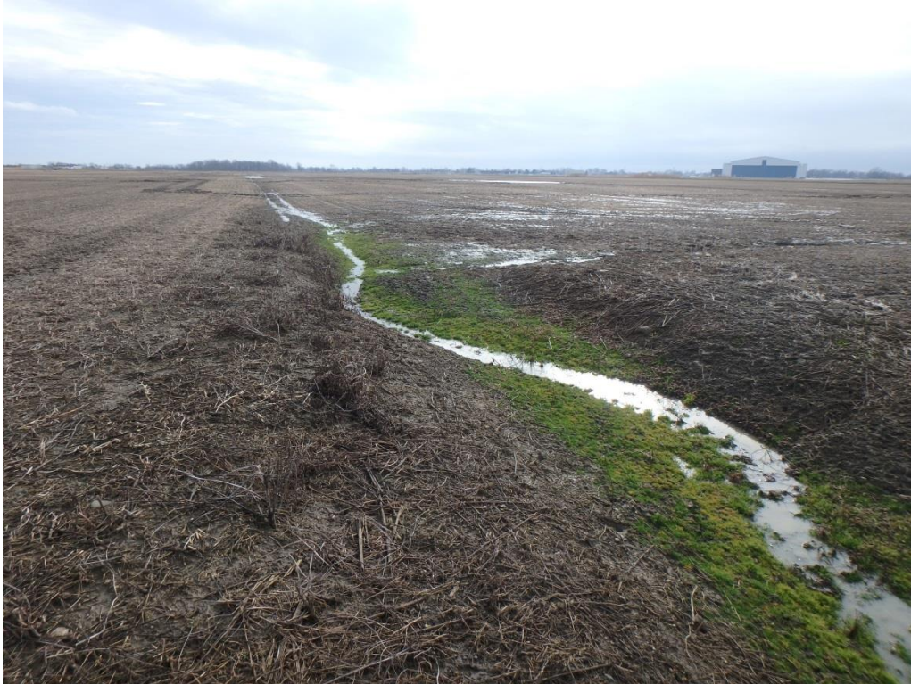
Photo 5 – Drainage Swale to Lappan Drain, Looking South
