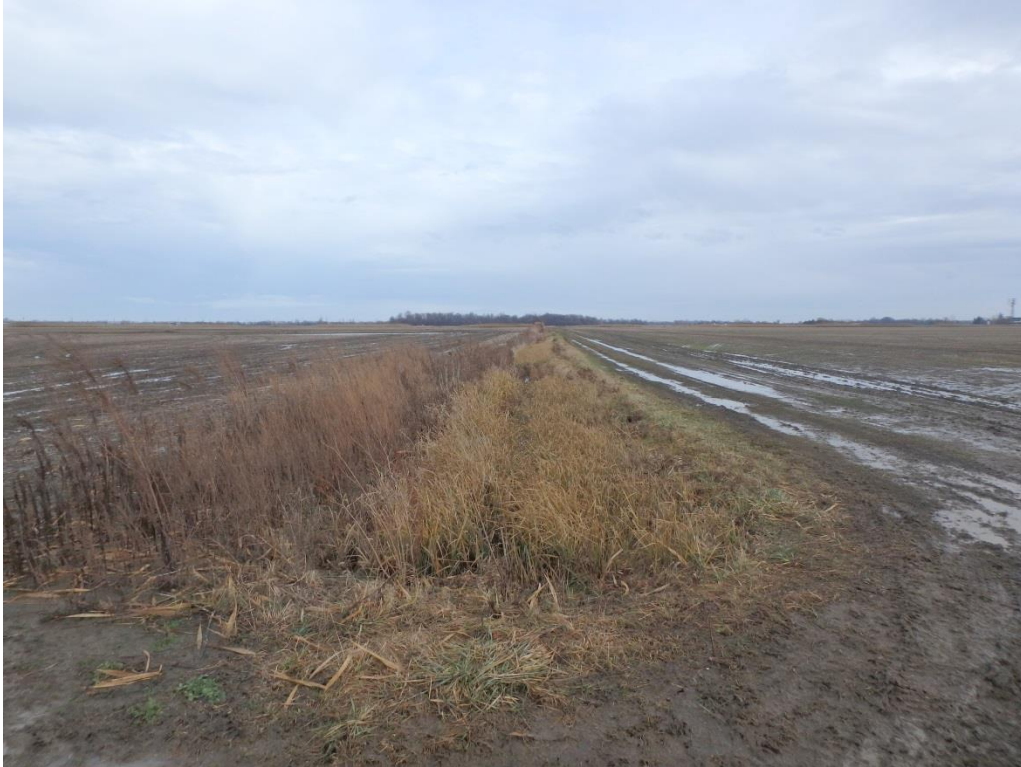
Photo 1 – McGill Drain at Pilette Road, Looking East
