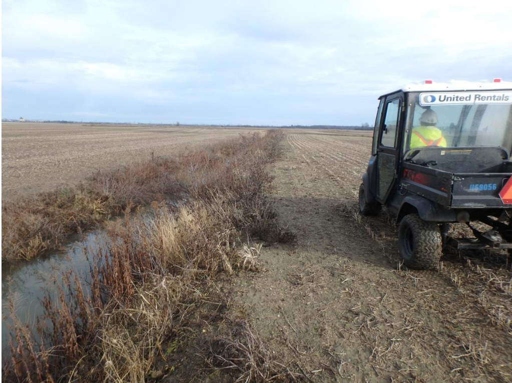
Photo 3 – Lappan Drain, Looking East
