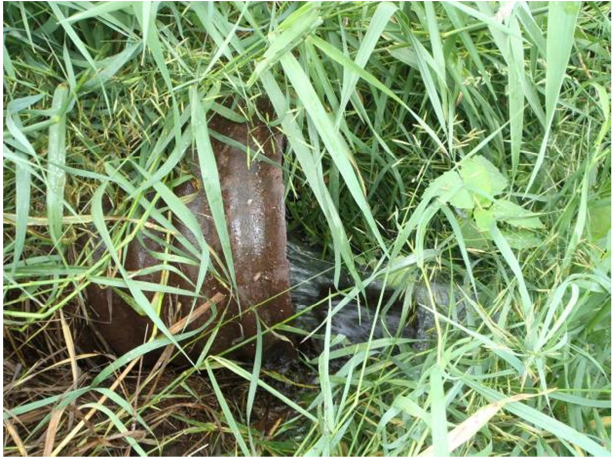
Photograph 41. Unnamed Stream 5 flowing through a CSP culvert crossing under the residential driveway.
