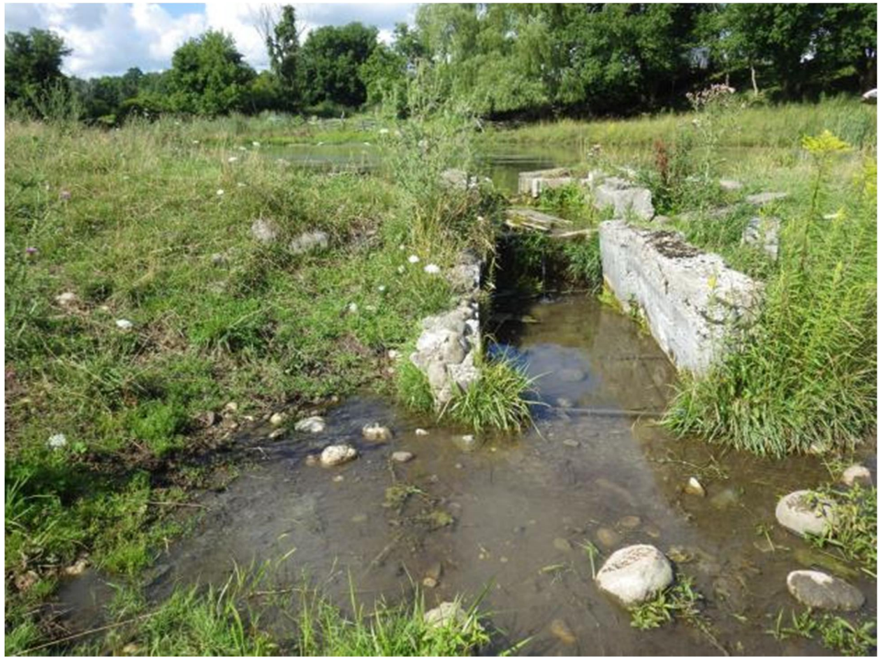
Photograph 29, facing northeast. Unnamed Stream 2 flowing from a dug pond and over a concrete weir.
