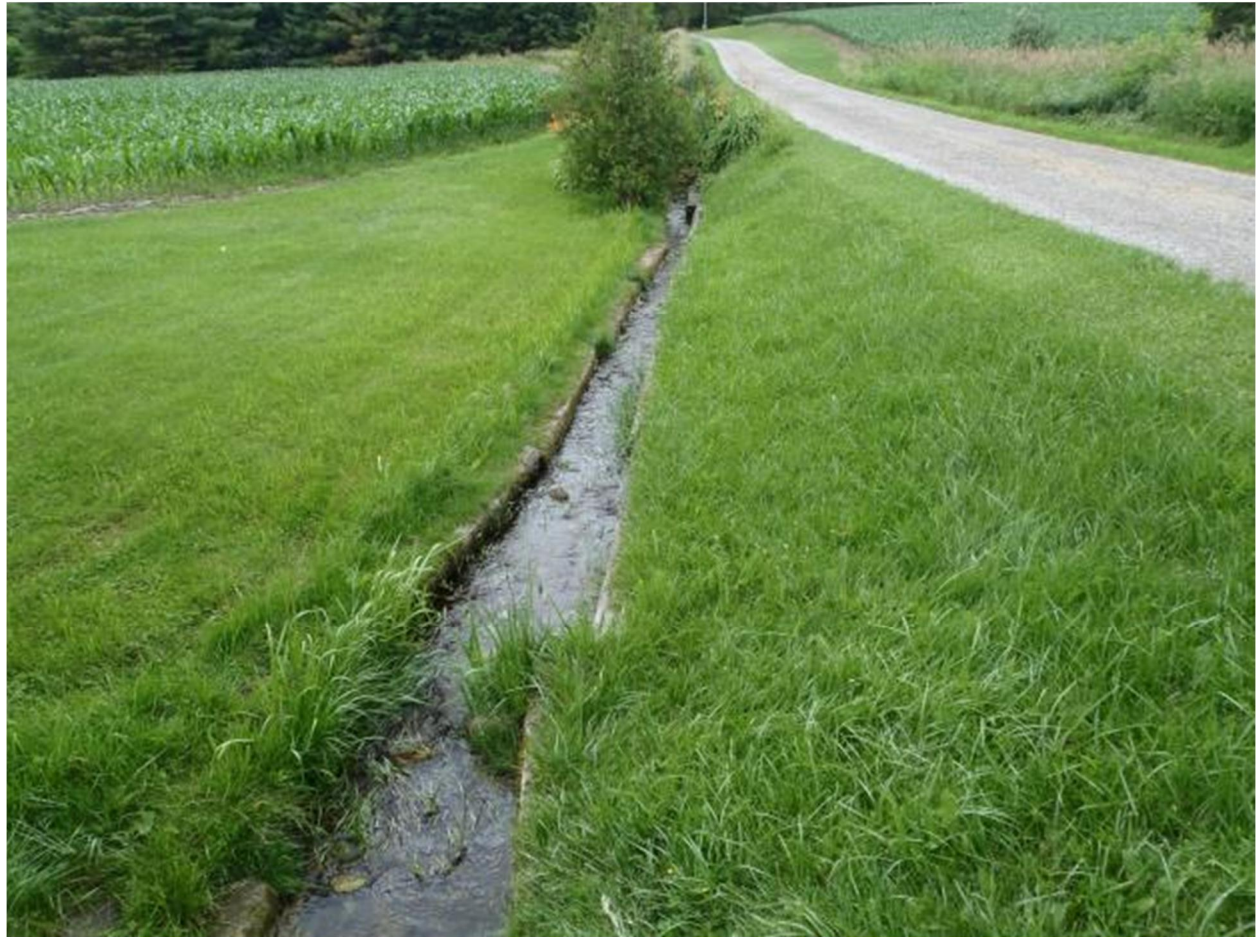
Photograph 39, facing west. Unnamed Stream 5 flowing west within a channelized ditch lined with concrete railroad ties on the south side of a residential driveway.
