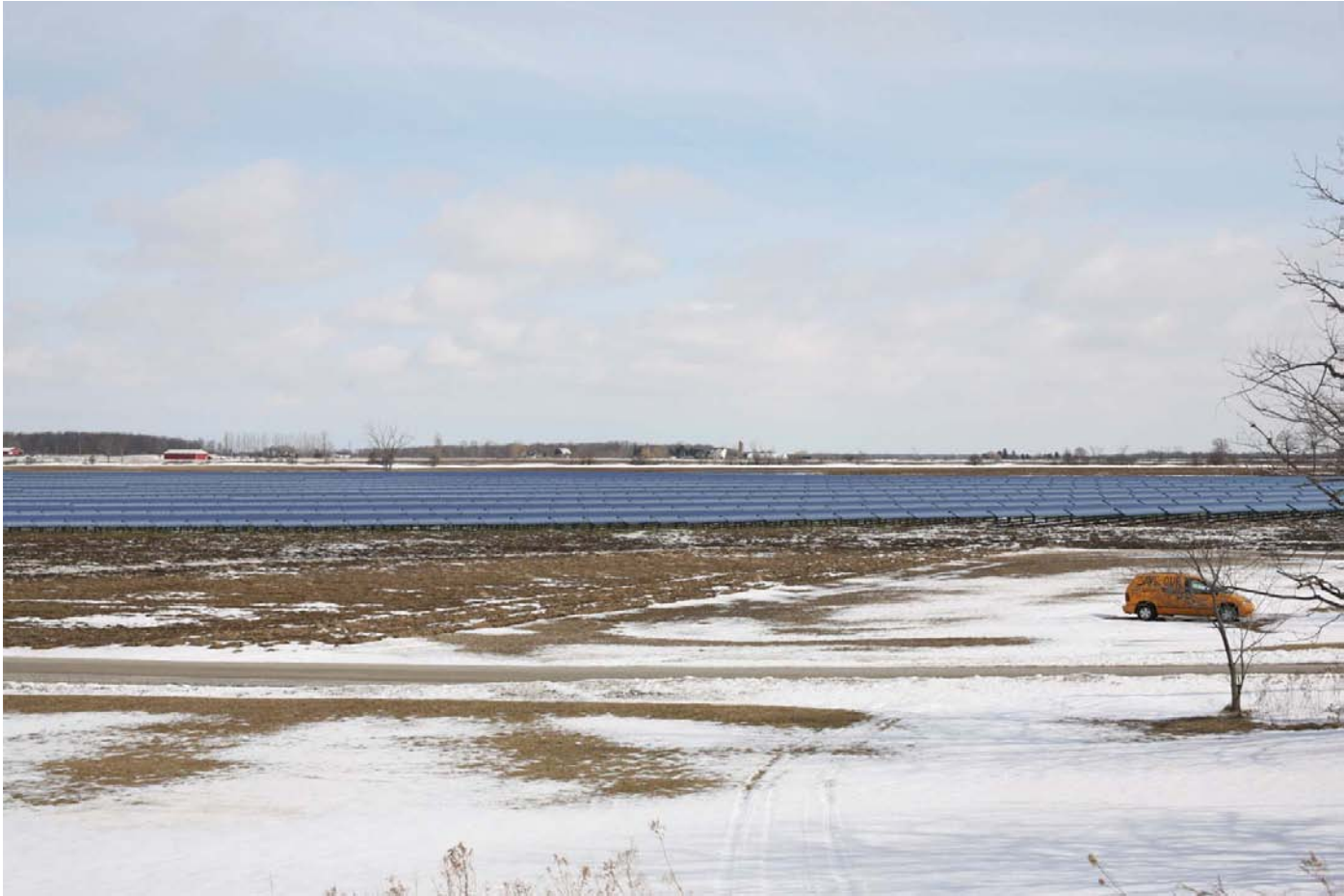
INSTALLATION OF SOLAR PANELS
