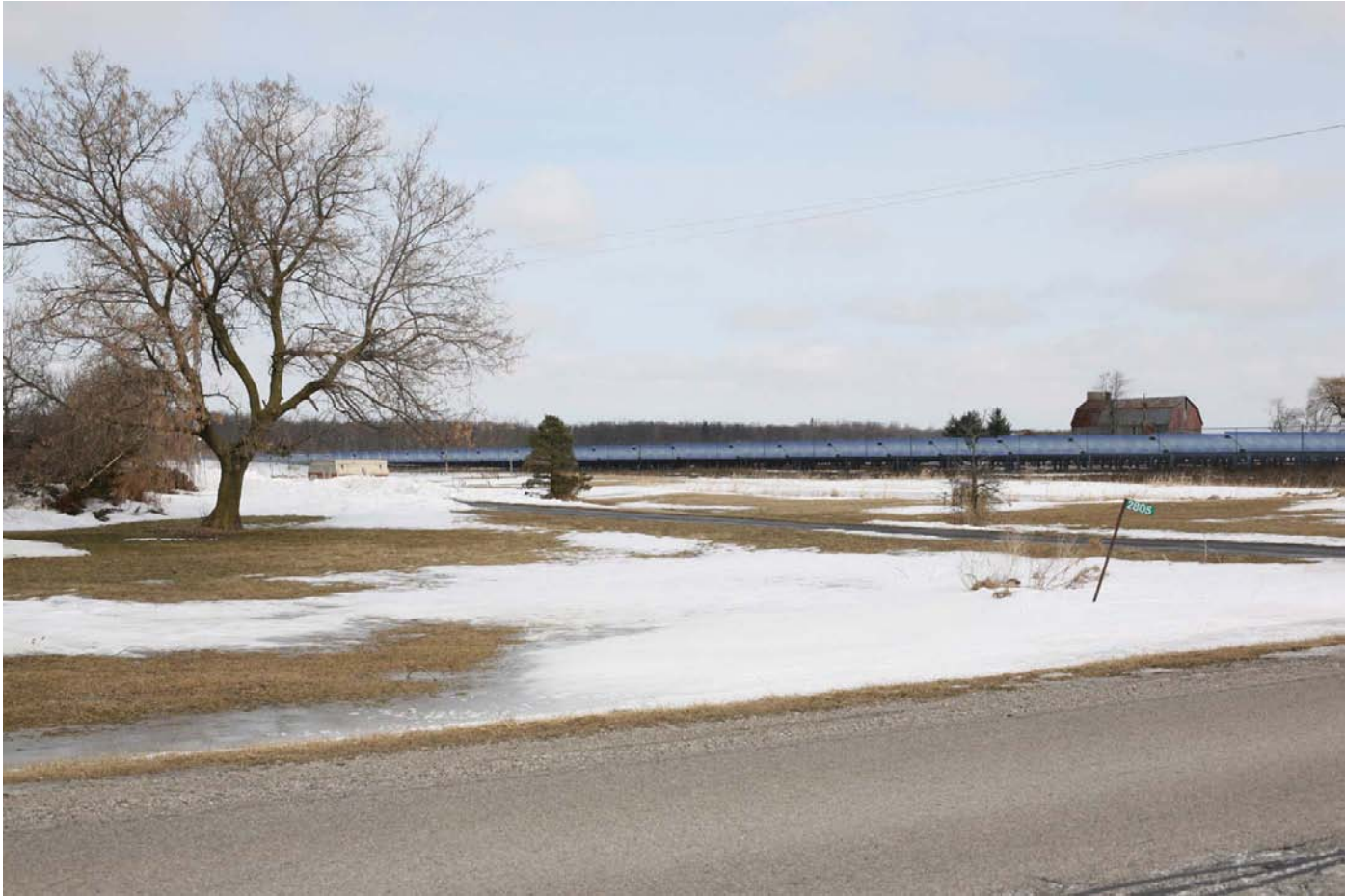
INSTALLATION OF SOLAR PANELS
