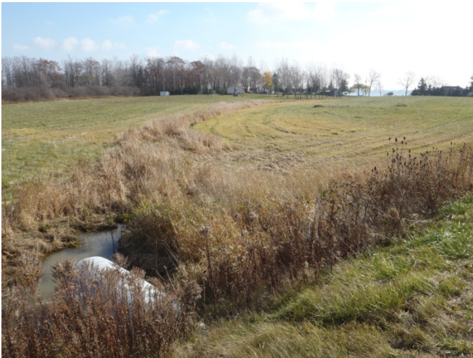
Photo 41: Lake-j (tile 10) - Looking downstream (southeast) at CSP culvert and water feature from Haldimand Road 50, approximately 300 m north of the lake shore.
