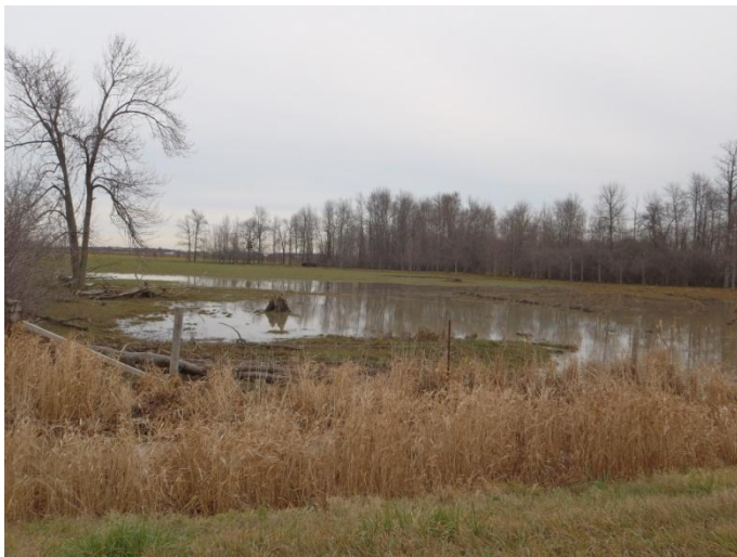
Photo 3: Ston-a (tile 19) - Looking upstream (northeast) from concrete culvert at flooded pasture. Site is located on Haldimand Road 20 between Concession 10 and Concession 11 W-1.
