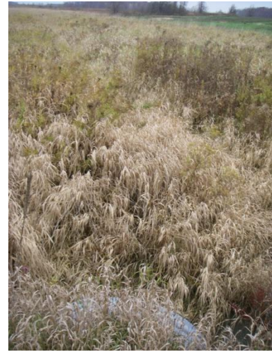
Photo 18: Ward-h (tile 9) - Looking upstream (northeast) at water body flowing from dense vegetation into CSP culvert. This site is located on Bains Road between Sutor Road and Haldimand Road 50.
