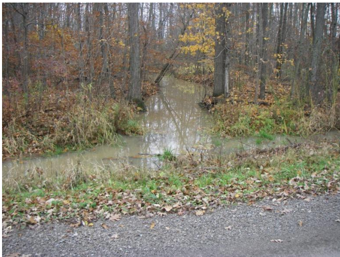
Photo 5: Hem-a (tile 4) - Looking north at confluence of roadside drain flowing west and channel flowing south through woodlot. This site is upstream of twin CSP culverts located on Concession 6 near the intersection of Haldimand Road 20.
