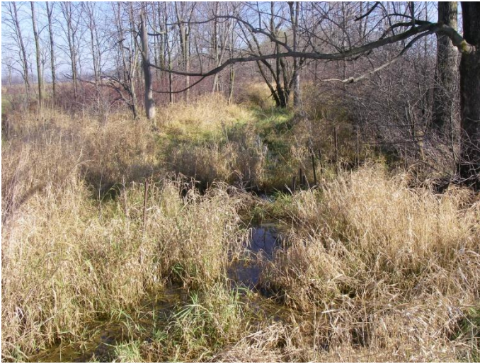
Photo 4: Ward-b (tile 6) - Looking upstream (south) from concrete culvert on Bains Road, between Haldimand Road 20 and Wilson Road.
