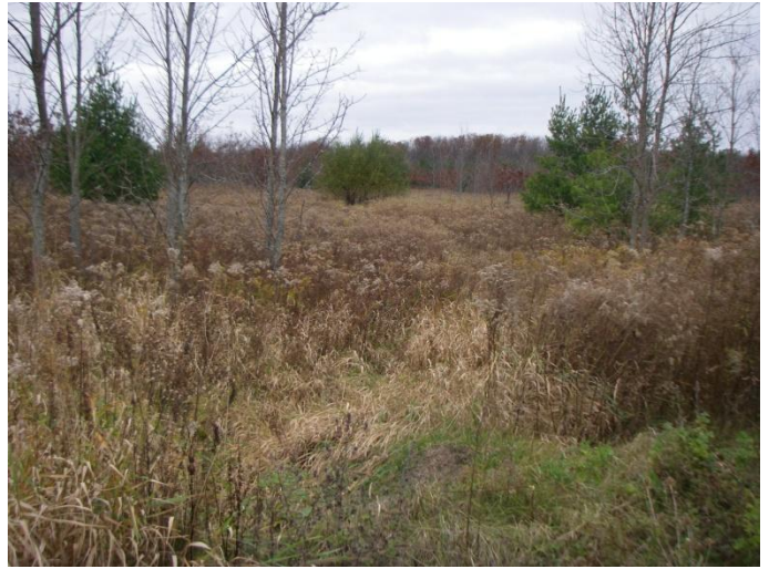
Photo 20: Ward-j (tile 8) - Looking upstream (northeast) at grassy swale from a CSP culvert in a field. Site is located west of Haldimand Road 50 between Haldimand Road 20 and Bains Road.
