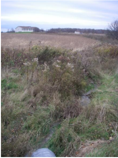
Photo 144: Evans-d (tile 12) - Looking at upstream (north) from CSP culvert flowing under Bains Road, south of Haldimand Road 20, between Haldimand Road 50 and South Cayuga Road.
