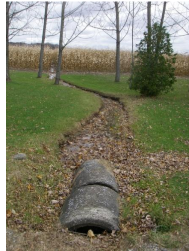
Photo 23: Hem-h (tile 4) - Looking downstream (east) from CSP culvert in laneway at linear channel flowing through a residential property. Note, channel flows through agriculture field downstream of residential property. Site is located west of Haldimand Road 20, between Concession 4 and Concession 5.
