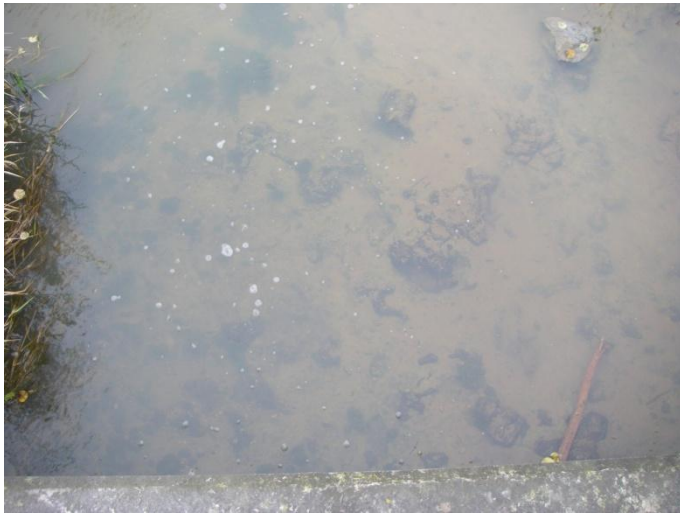
Photo 14: Ward-f (tile 8) - Existing substrate conditions in water body at downstream end of concrete culvert. This site is located on Bains Road between Wilson Road and Haldimand Road 50.
