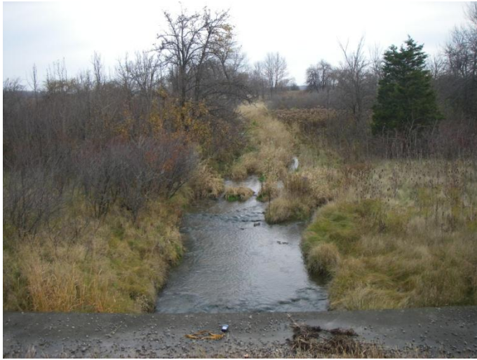
Photo 12: Ward-f (tile 8) - Looking upstream (northwest) at water body flowing into a concrete culvert. This site is located on Bains Road between Wilson Road and Haldimand Road 50.
