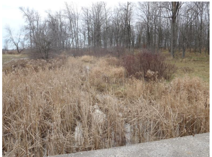
Photo 4: Ston-a (tile 19) - Looking downstream (southwest) from concrete culvert at flooded vegetation. Site is located on Haldimand Road 20 between Concession 10 and Concession 11 W-1.
