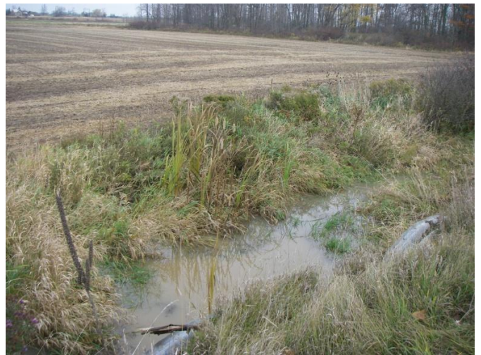
Photo 6: Hem-a (tile 4) - Looking west at roadside drain flowing into Water Body on south end of twin CSP culverts located on Concession 6 near the intersection of Haldimand Road 20.
