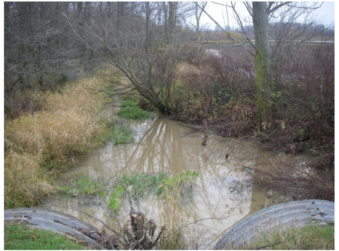
Photo 2: Hem-a (tile 4) - Looking downstream (south) at Water Body and twin CSP culverts located on Concession 6 near the intersection of Haldimand Road 20. Note flooded agricultural fields on west bank and woodlot on east bank.
