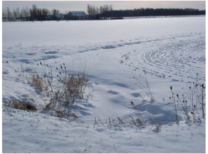
Photo 41: Hem-m (tile 6) - Looking downstream (southwest) at roadside drain and channel flowing through an agricultural field. Site is located on Kohler Road between Concession 4 and Concession 5.
