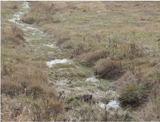
Photo 19: Ston-f (tile 18) - Existing substrate conditions downstream of concrete culvert. Site is located on Haldimand Road 20 between Dry Lake Road and Highway 3.
