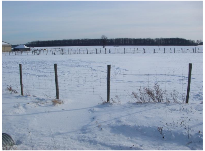
Photo 44: Hem-n (tile 6) - Looking south at outflow of CSP culvert into pasture lands. Site is located on Concession 4, between Kohler Road and Haldimand Road 20.
