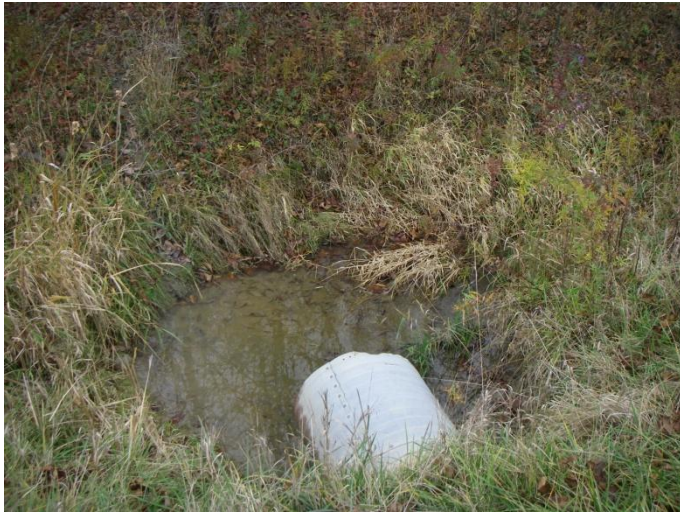
Photo 11: Hem-c (tile 4) - Looking downstream (west) at small pool in roadside drain associated with CSP culvert. This site is on Haldimand Road 20 between Concession 5 and Concession 6.
