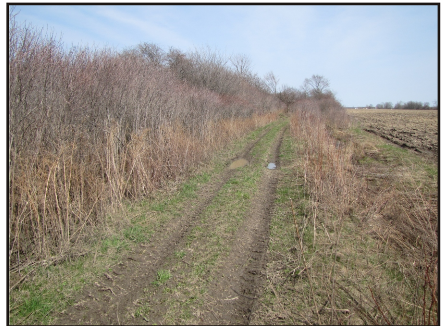
Photo 8 - Looking East Along Ramsay Road RoW Between Turbine Complex 3 Access Road and T64
