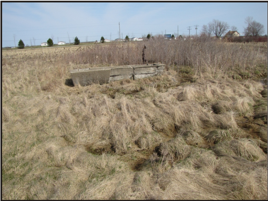
Photo 15 - Water Trough, Looking East From North Side of Foundation 1
