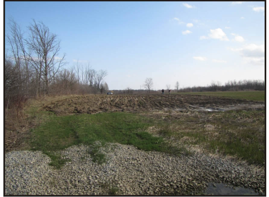
Photo 6 - Turbine 58 Access Road, Looking South From Watercourse to Road
