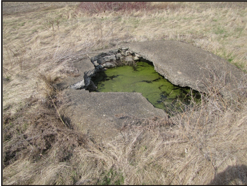
Photo 13 - "Well" Feature Between Foundations at Incinerator
