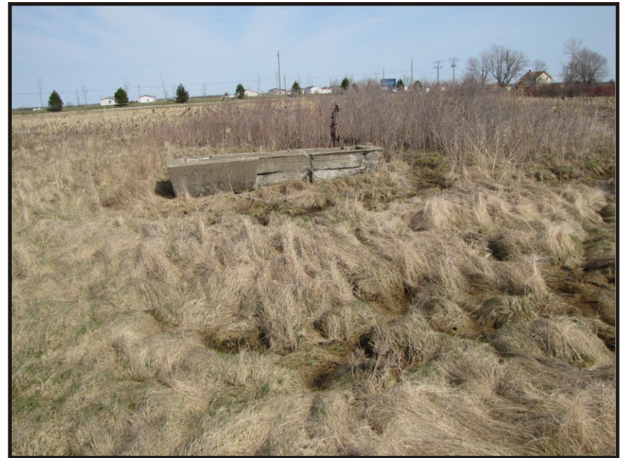
Photo 12 - Water Trough, Looking East From North Side of Foundation 1
