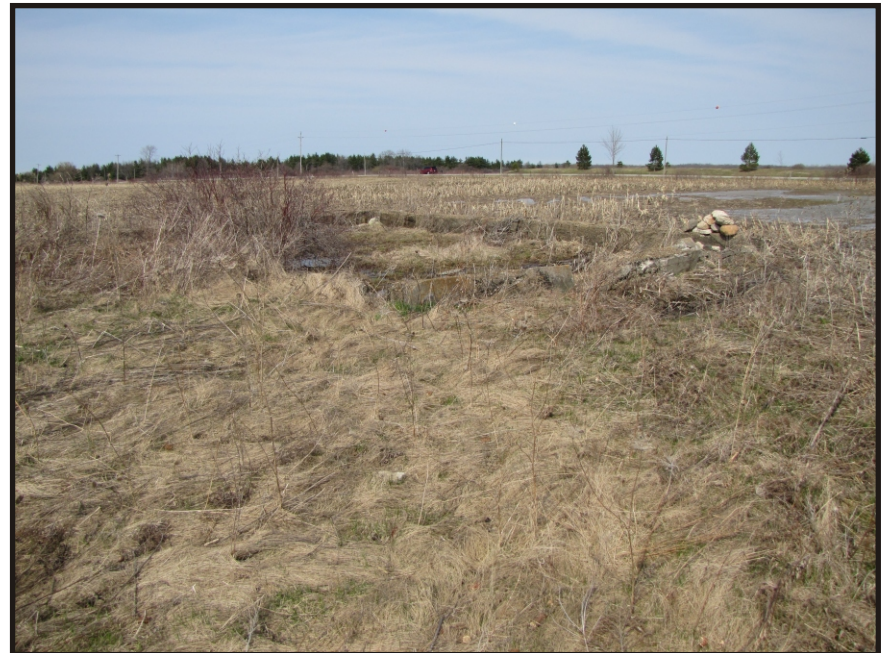
Photo 14 - Foundation 2, North-East Corner, Looking From South
