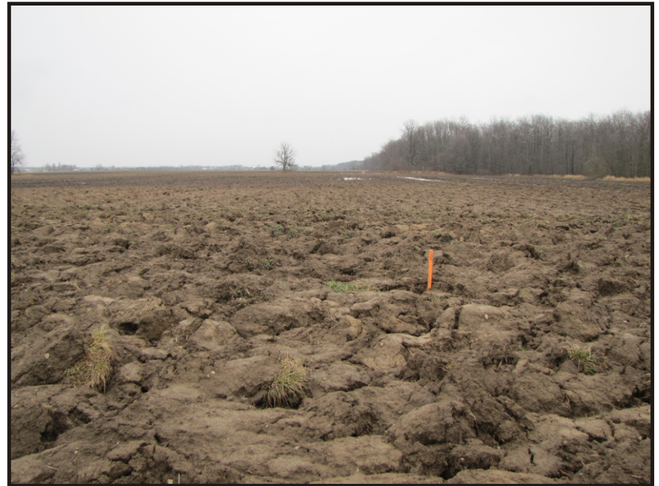
Photo 8 Stake Marking Centrelines for Turbine Access Roads in Ploughed Fields
