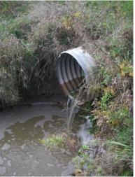
Photo 81: Gran-z (tile 11) - Looking at perched CSP culvert on east side of South Cayuga Road. This site is located on South Cayuga Road between Haldimand Road 20 and Bains Road.
