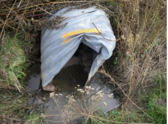
Photo 79: Gran-z (tile 11) - Looking at damaged CSP culvert on west side of South Cayuga Road. This site is located on South Cayuga Road between Haldimand Road 20 and Bains Road.
