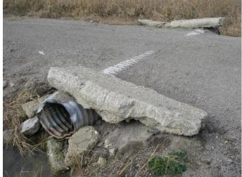
Photo 41: Gran-j (tile 5) - Looking at downstream end of perched CSP culvert in laneway at ephemeral feature that flows through an agricultural field. Site is located east of Haldimand Road 20, between Richert Road and Kohler Road.
