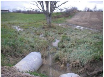
Photo 100: Gran-ee (tile 13) Looking upstream (west) at twin CSP culverts and standing water from farm access road. Site is located north of Haldimand Road 20 between Hald-Dunn Townline Road and Old Hines Road.
