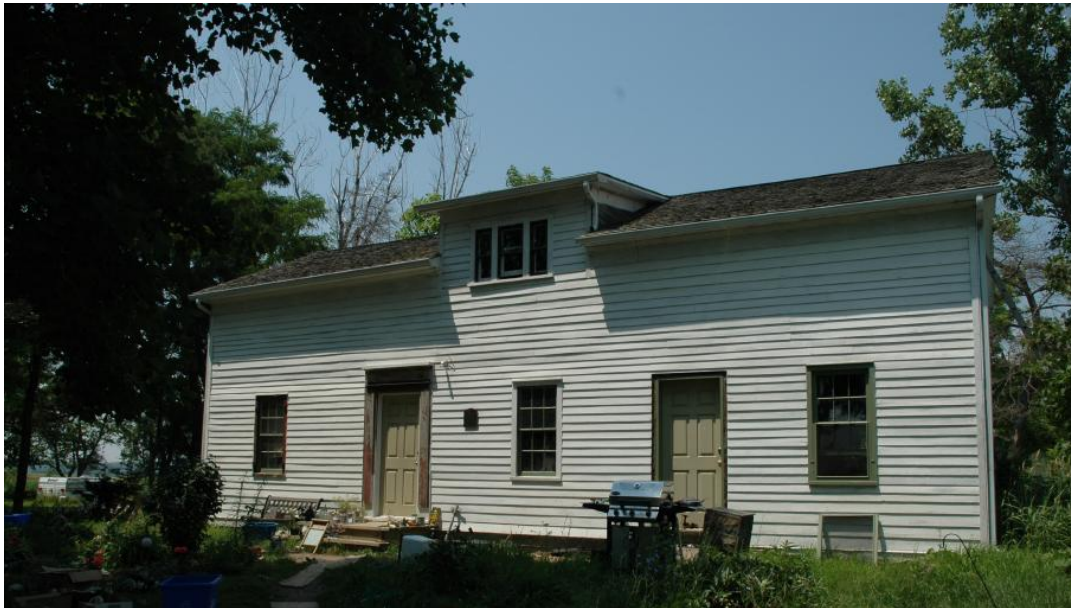
Photograph 7 - The John Fry House, front elevation, facing north
