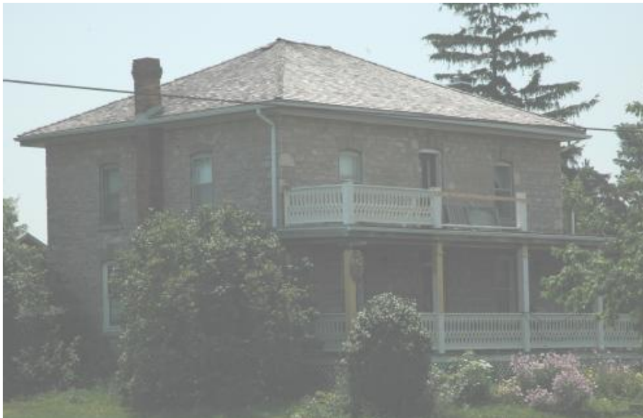
Photograph 1 - The Campbell-Pine House, front elevation, facing southwest.
