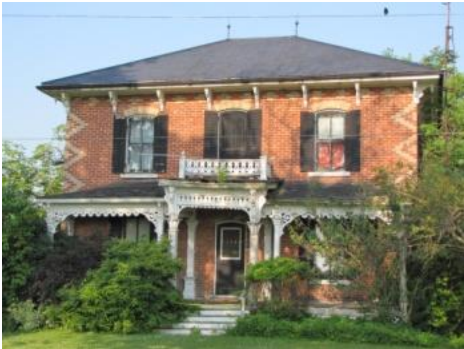
Photograph 5 - The Charles Reicheld House, front elevation, facing east
