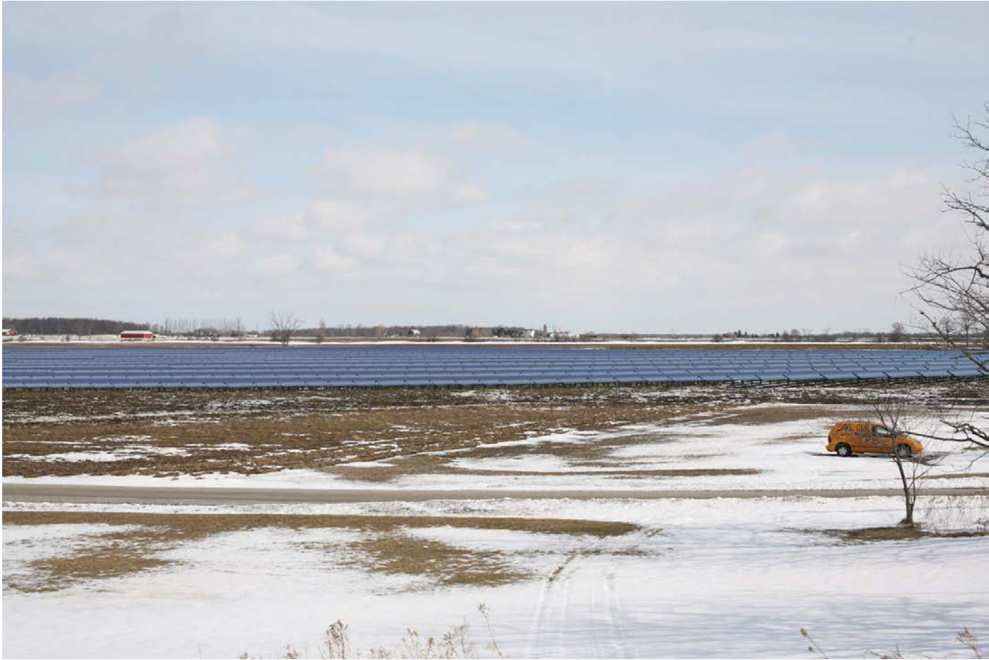
INSTALLATION OF SOLAR PANELS
