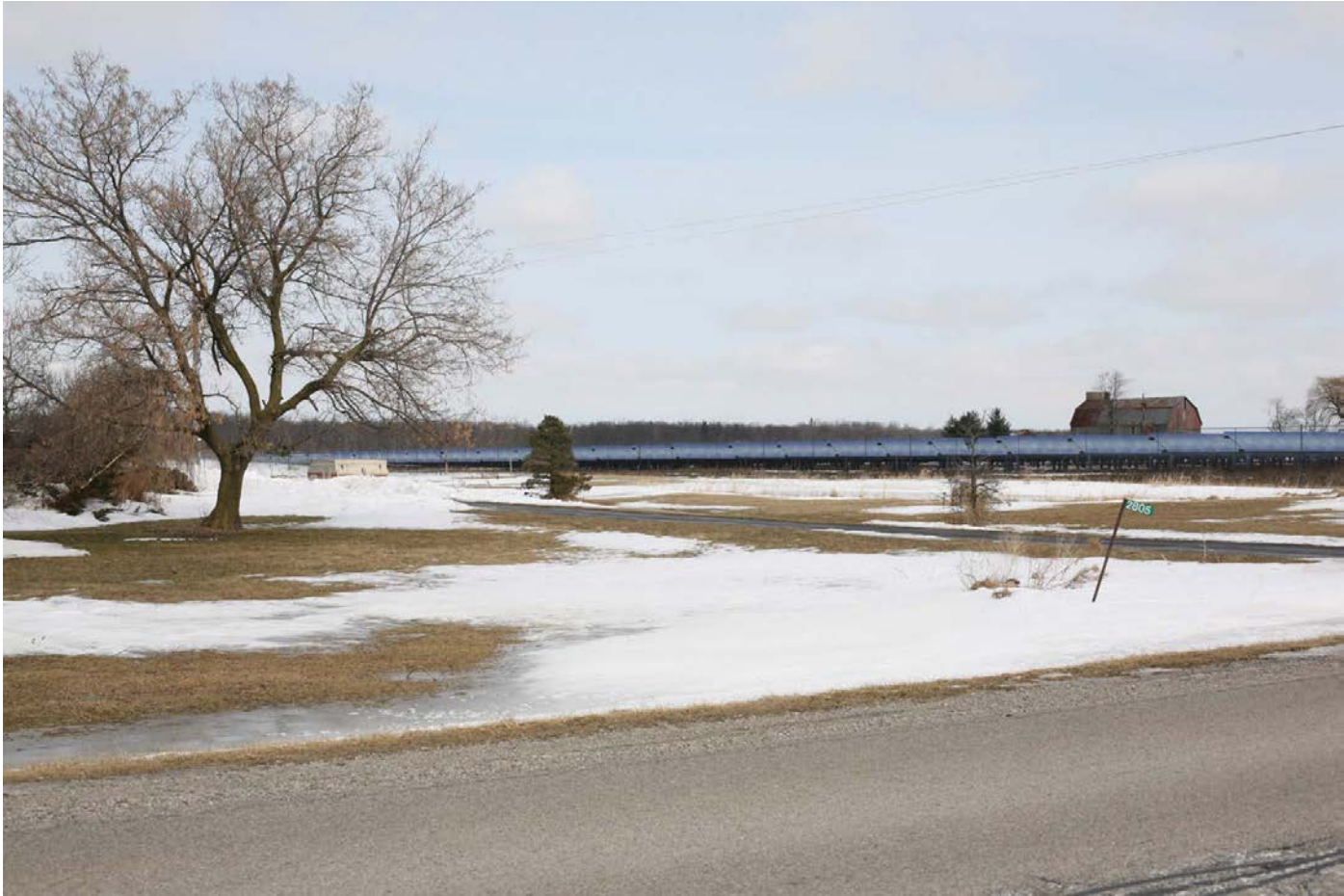
INSTALLATION OF SOLAR PANELS
