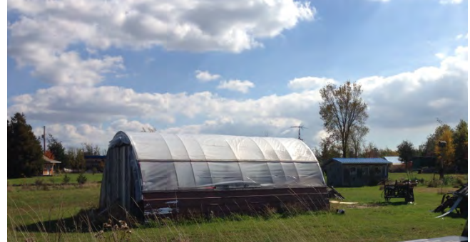
Plate 2 Property 2, looking east, various outbuildings (outside Project Location)
