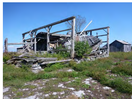
Plate 4 Property 25A, looking northeast, barn ruins
