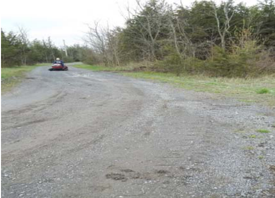
Photograph 1: View of gravel covered roadway within Parcel 1-2, facing southwest.
