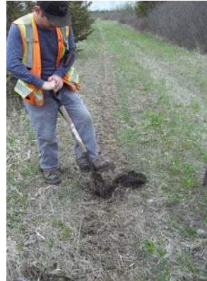
Photograph 16: View of test-pitting program in grass covered access road within Parcel 1-2, facing east.
