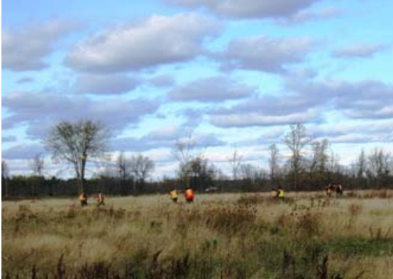
Photograph 103: View of AMEC personnel conducting test-pitting program within Parcel 14B, facing north.
