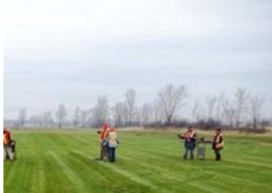
Photograph 106: View of AMEC personnel conducting test-pitting program within Parcel 14C, facing north.
