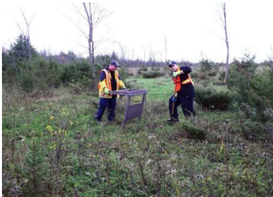
Photograph 89: View of AMEC personnel conducting test-pitting program within Parcel 13, facing southwest.
