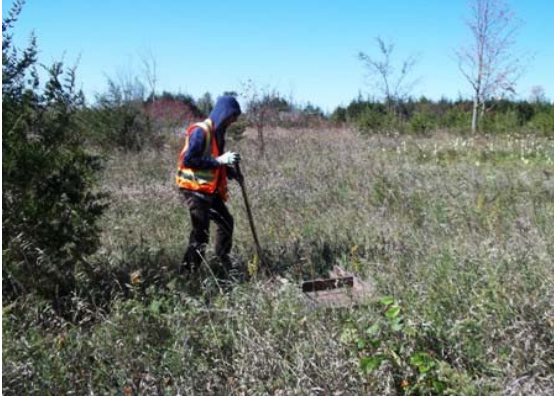
Photograph 49: View of AMEC personnel conducting test-pitting program within Parcel 1, facing south.
