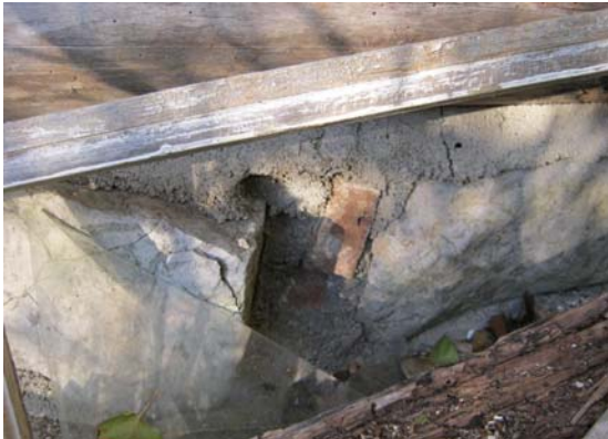
Photograph 153: View of historic foundation associated with BbGd-50, facing north. Note modern brick and cement within foundation.
