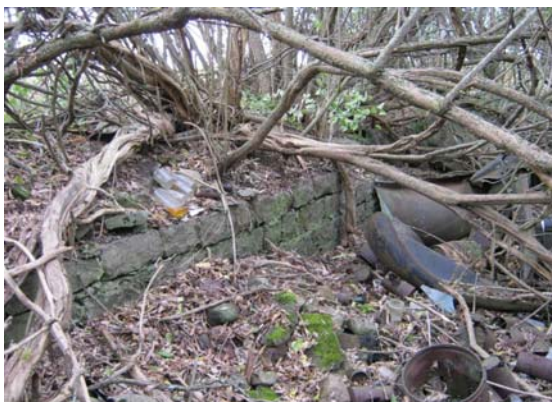
Photograph 137: View of historic foundation associated with BbGd-49, facing east.
