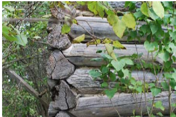
Detail of V-notched round logs and chinking of derelict log structure.
