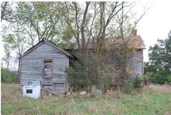
View of the rear and the north side of the structure.
