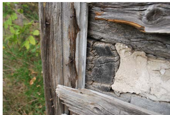
Detail of the iron nails and chinking.
