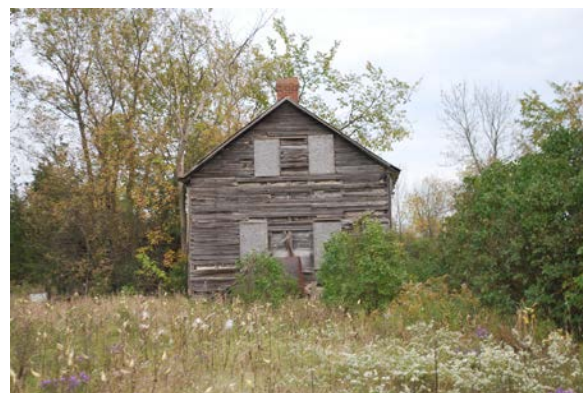
View of the east side of the structure.
