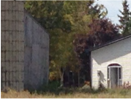
Plate 13 Property 25B, looking southwest, foliage coverage of residence (outside Project Location)
