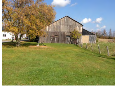
Plate 14 Property 25B, looking north, timber barn (outside Project Location)
