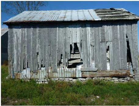
Plate 7 Property 25A, looking north, outbuilding
