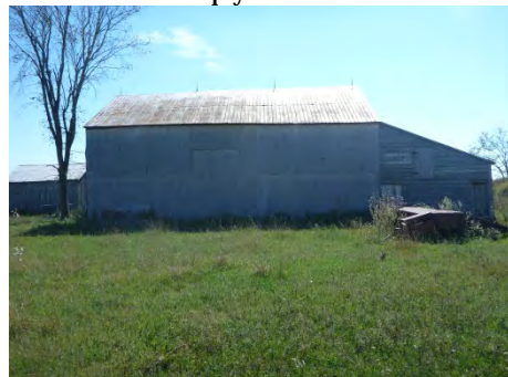
Plate 6 Property 25A, looking south, timber barn clad in plywood
