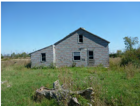
Plate 9 Property 25A, looking east, residence
