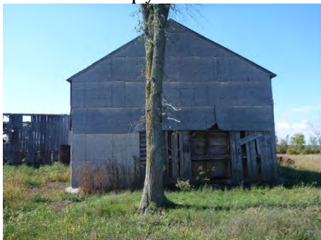
Plate 5 Property 25A, looking west, timber barn clad in plywood
