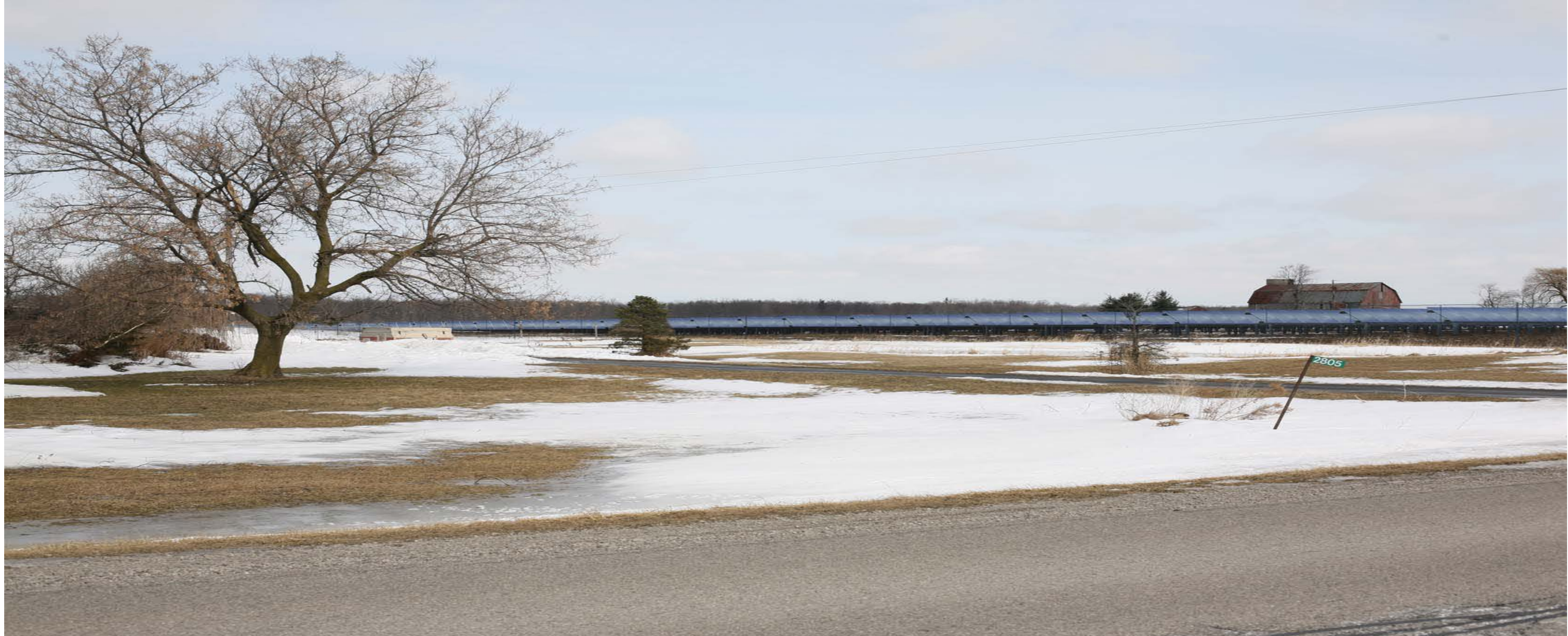
INSTALLATION OF SOLAR PANELS
