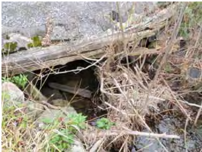
Photo 35: Glenvale Cr. Trib.2c culvert has pooled water present but no water upstream or downstream in suspected seasonal swale between fields. Site ID# P6A-1
