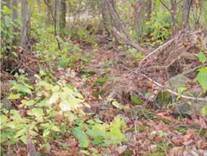
Photo 1: Looking south towards Rock Rd. culvert on Glenvale Cr. Trib.1. Intermittent drainage is diffuse upstream to downstream culvert. Site ID# P1-A
