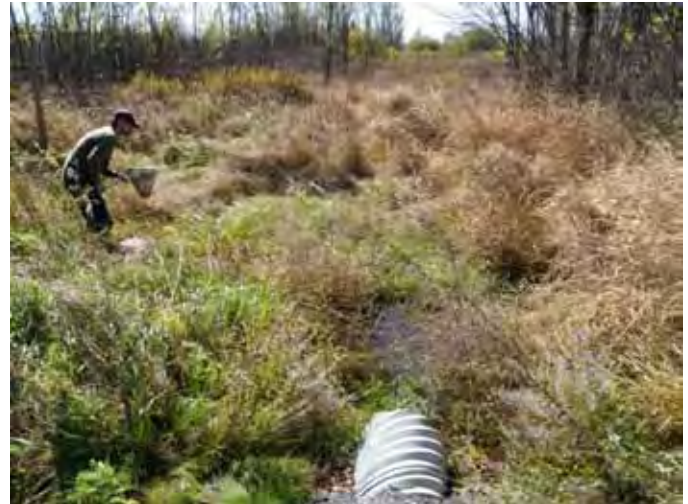
Photo 66: Looking west from Hegadorn Rd. laneway CSP with diffuse pooled pockets of water ~0.10m deep with no defined channel. ID# P24-D
