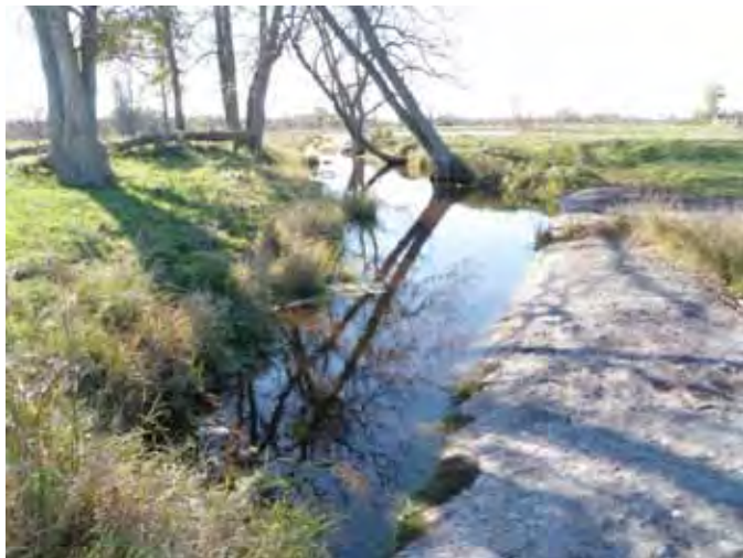
Photo 91: Looking south at dug out permanent drainage feature from fields on north side (Property 6A) of Unity Rd. Site ID# P14-B1
