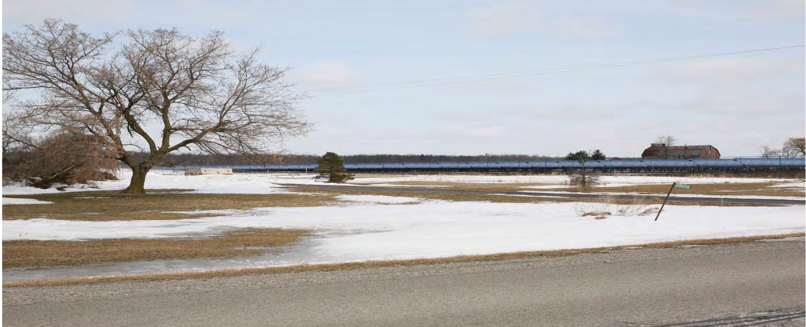
INSTALLATION OF SOLAR PANELS
